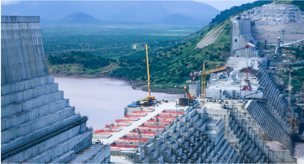
Ethiopia's Grand Renaissance Dam is seen as it undergoes construction work on the river Nile in Guba Woreda, Benishangul Gumuz Region, Ethiopia September 26, 2019. Picture taken September 26, 2019. Tiksa Negeri/Reuters.
